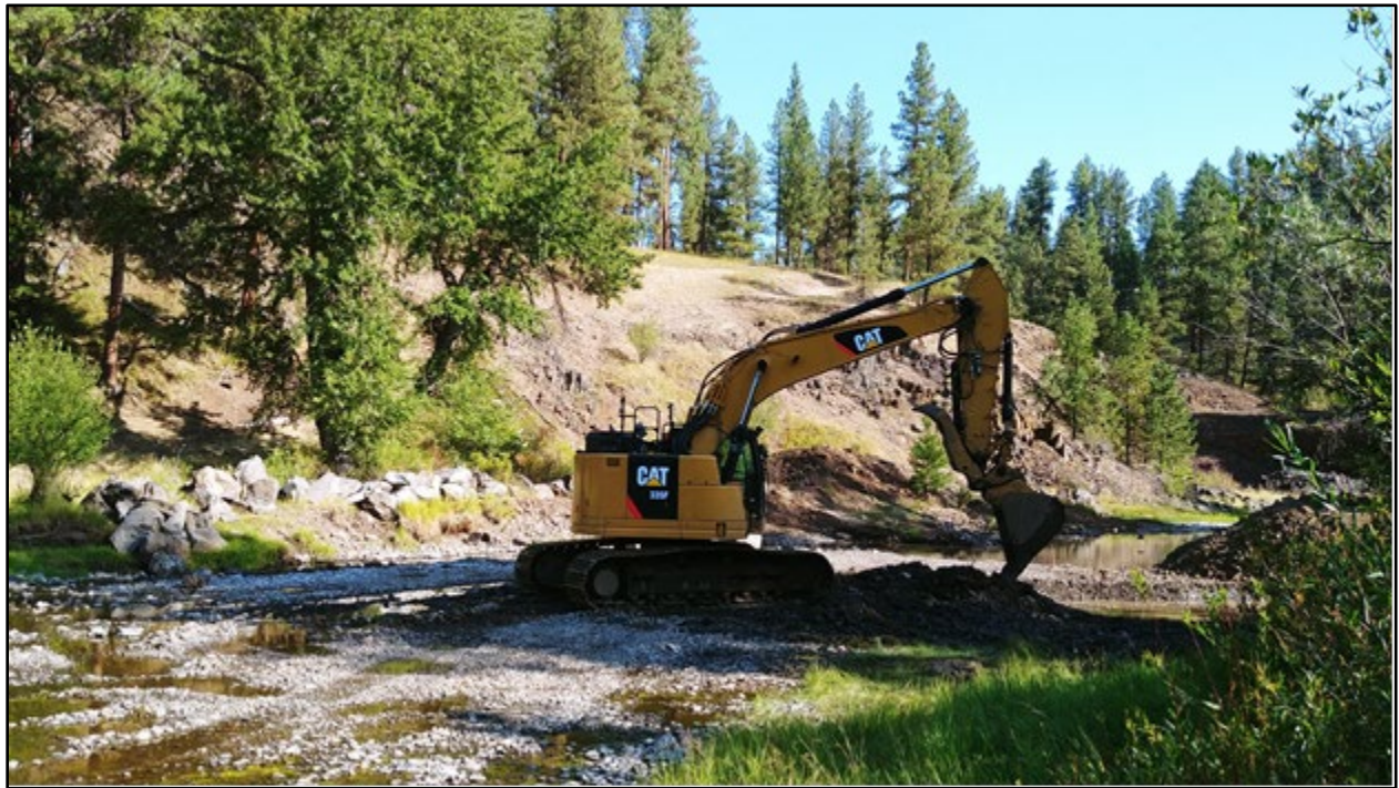
FIGURE 22 MAIN CHANNEL RIFFLE AND SIDE CHANNEL ENTRANCE CONSTRUCTION
