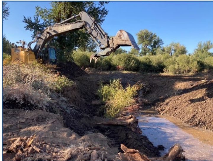
FIGURE 5 REPLANTING SALVAGED WILLOW CLUMPS, LONGLEY MEADOWS PROJECT
